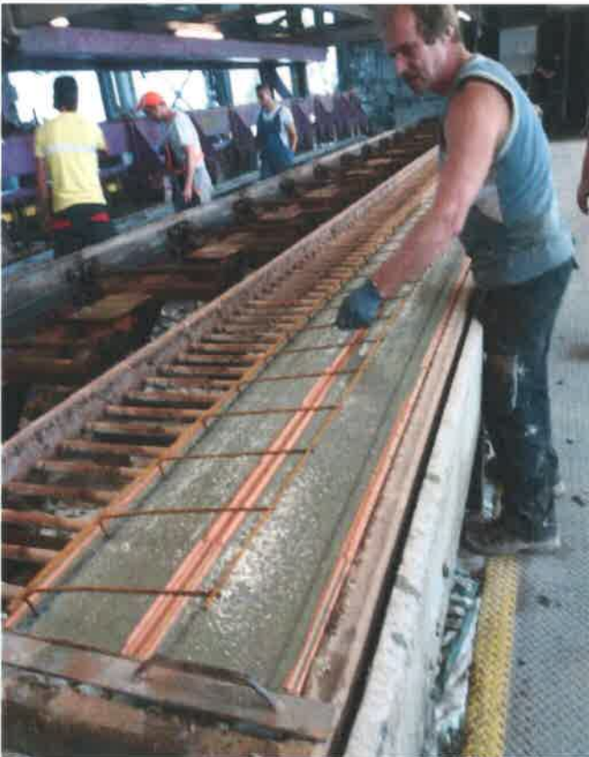
Photo 4 – Inserting steel reinforcement
