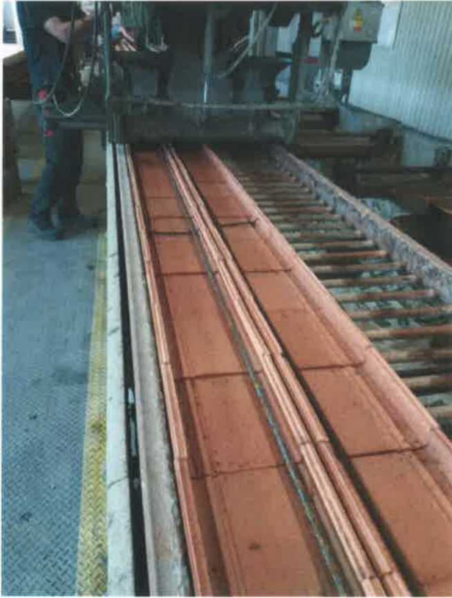
Photo 2 – Moistured U-shaped masonry units before concrete placement
