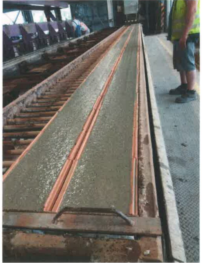
Photo 3 - U-shaped masonry units after concrete placement
