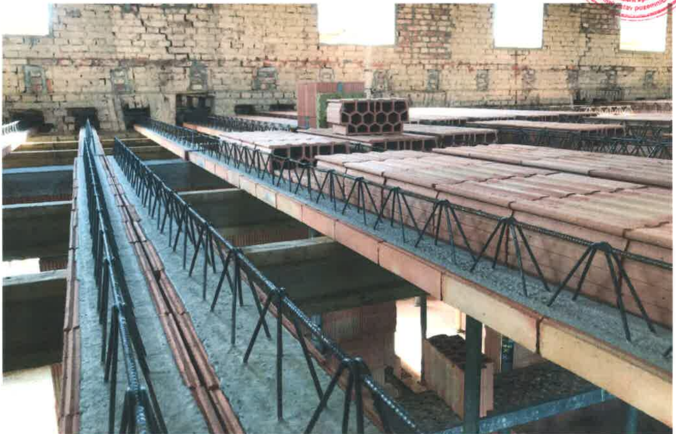
Photo 7 – Ceiling beams POT used for building reconstruction
