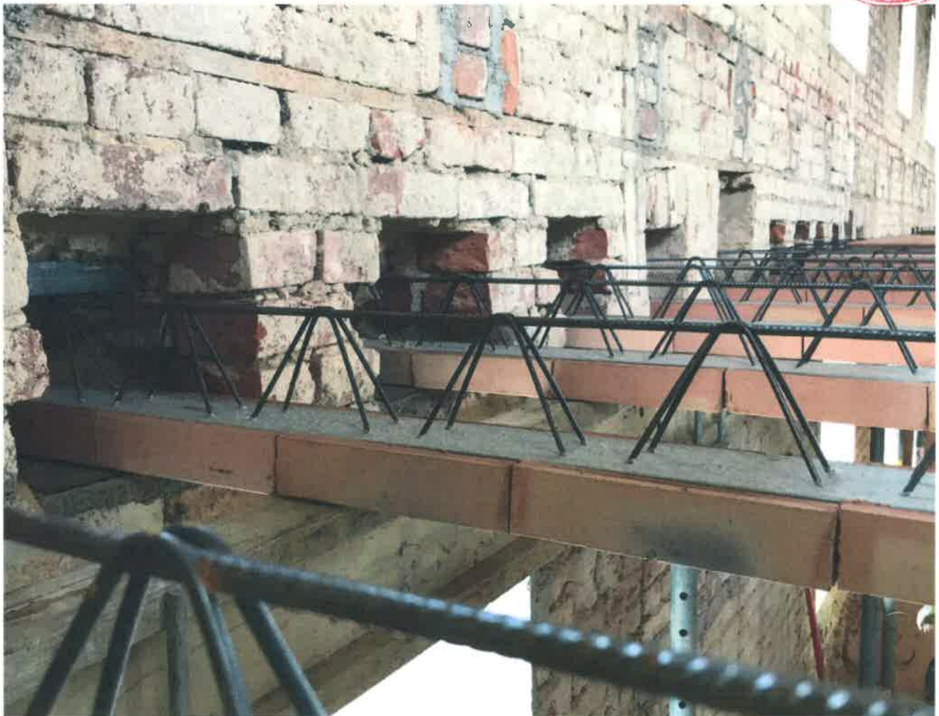
Photo 8 – Ceiling beams POT used for building reconstruction
