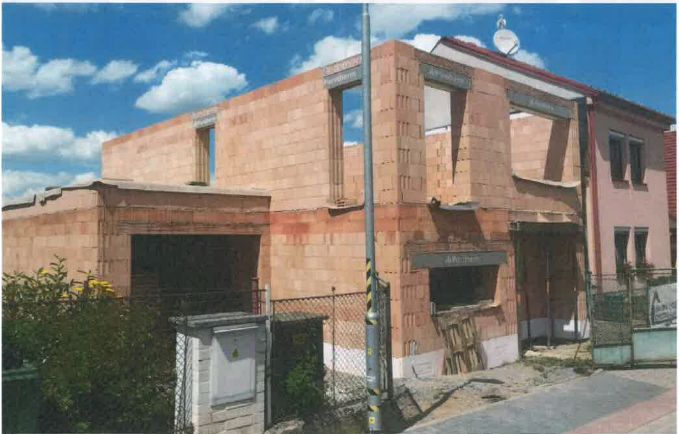
Photo 6 – Built-in KP Vario UNI lintels
