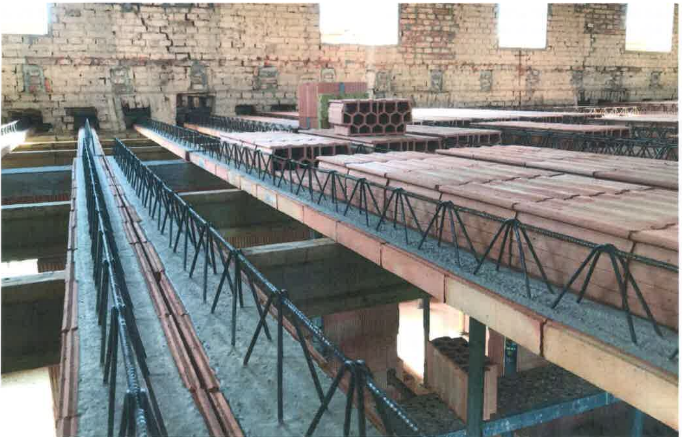
Photo 7 – Ceiling beams POT used for building reconstruction
