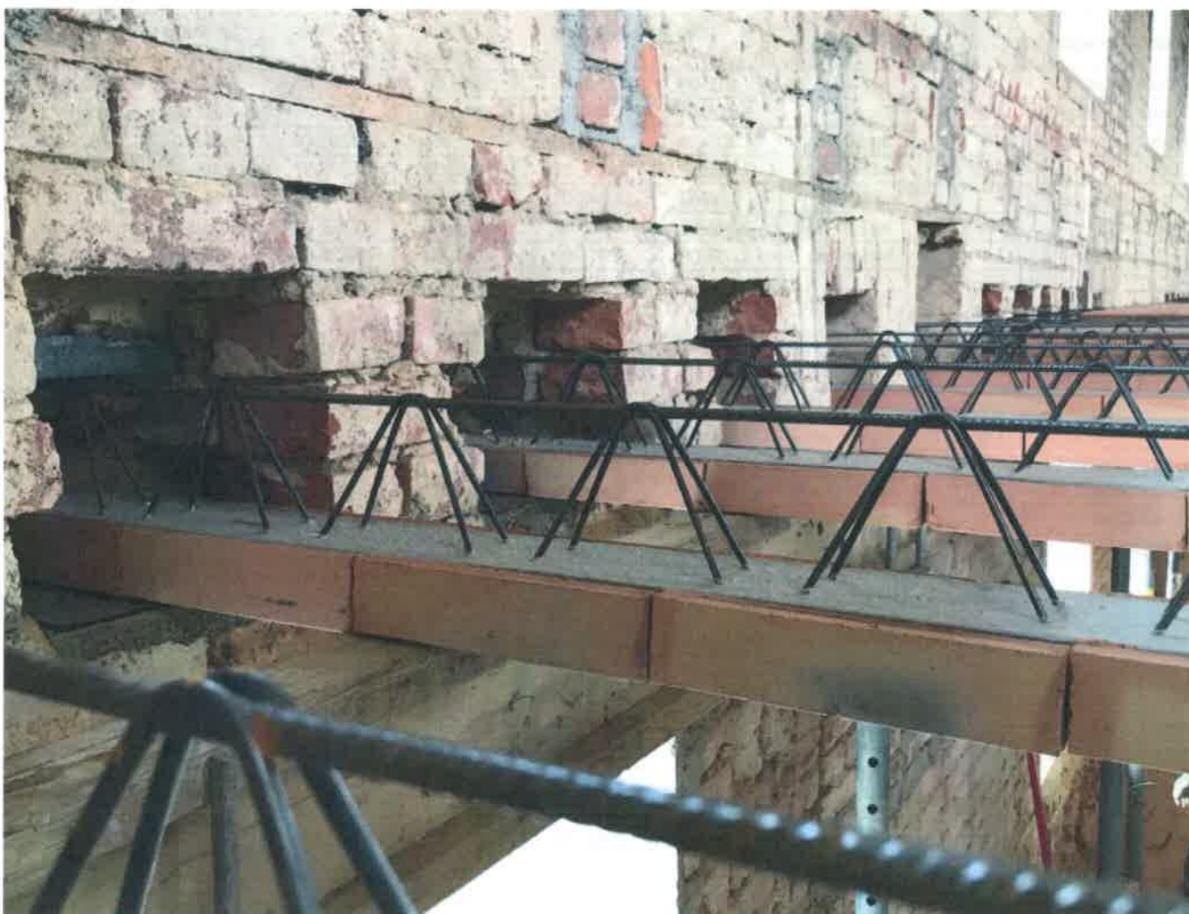
Photo 8 – Ceiling beams POT used for building reconstruction
