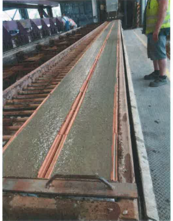
Photo 3 - U-shaped masonry units after concrete placement
