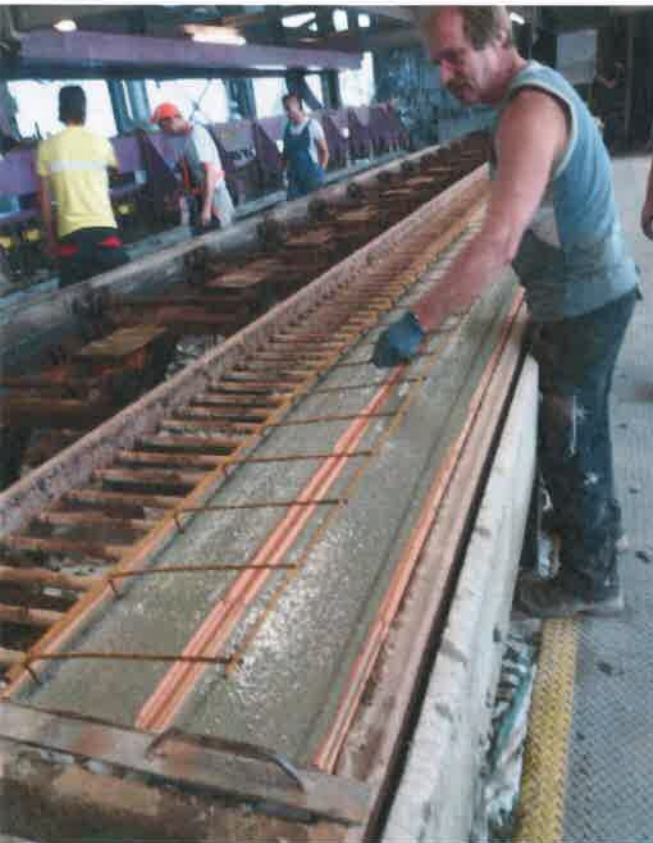
Photo 4 – Inserting steel reinforcement
