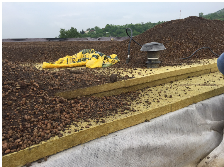
Fig. 1 - Example of CA 514 application
