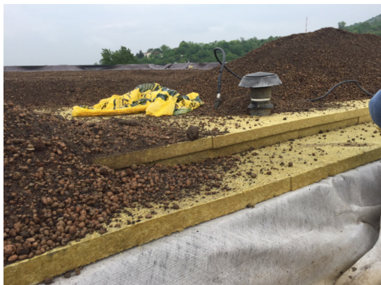
Fig. 1 - Example of CA 507 application
