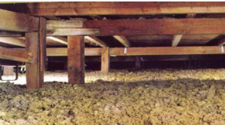
Fig. 5 - Blown insulation
