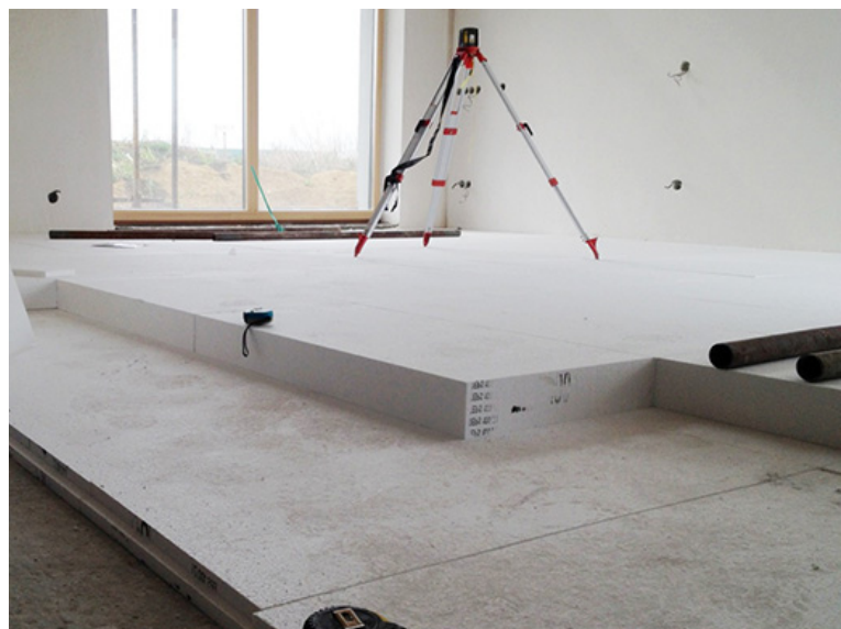
Fig. 1 - Example of Isover EPS 150 application
